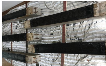
(c) Finished RC beams reinforcement.
