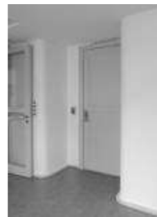
Plastered walls with rounded corners.
