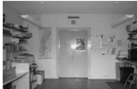
Room 609 to the west (corridor). Typical door lining.
