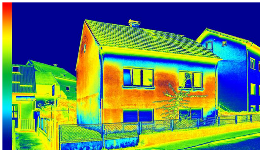
Figure 13: Heat photo of a house (Milieu Centraal, 2022)
