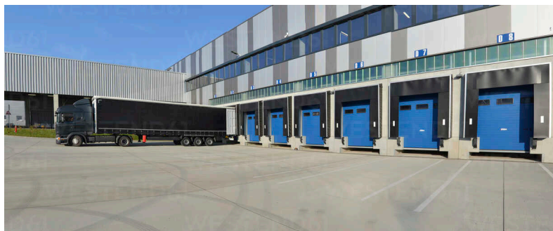
Figure 1.1: Dock door system (loading bay) (Lyzs, 2022)
