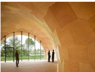
Figure [D2] [Forstpavilion] Reprinted from Itke website, by Roland Halbe, retrieved from https://www.itke.uni-stuttgart.de/de/archives/portfolio-type/landesgartenschau
