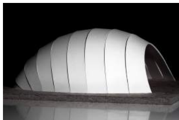
Figure [D3] [Bending active segmented shell] Reprinted from Itke website, retrieved from https://www.itke.uni-stuttgart.de/de/archives/portfolio-type/bending-active-segmented-shells
