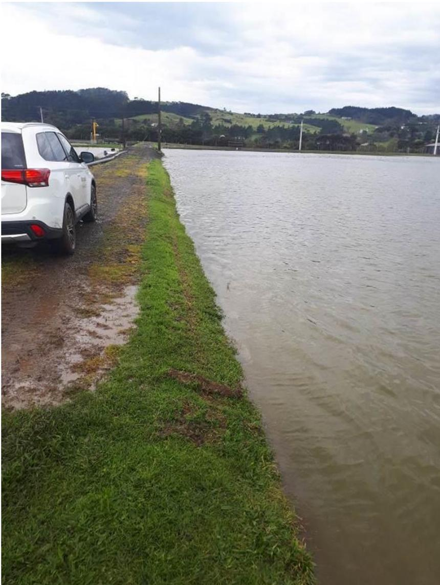
Figure 2: 9<sup>th</sup> September 2017 wet weather event (125mm between 3<sup>rd</sup> and 11<sup>th</sup> Sep). Pond levels at 1660mm. The pond will overtop the dam embankment into the harbour at 1.85m.
