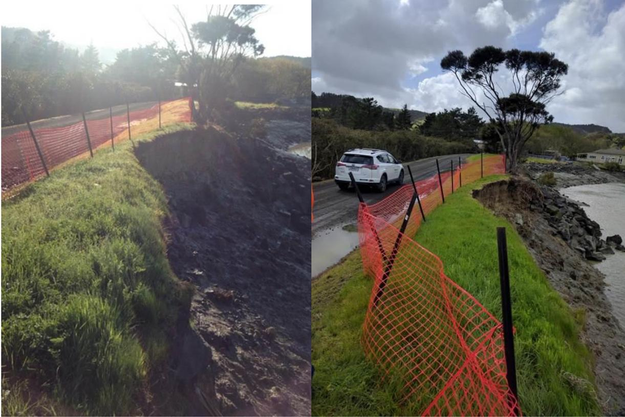
Figure 2: Access road erosion on the 9<sup>th</sup> September and 3<sup>rd</sup> October 2019. Approximately 0.5m erosion since the previous picture taken on 21st March 2019.
