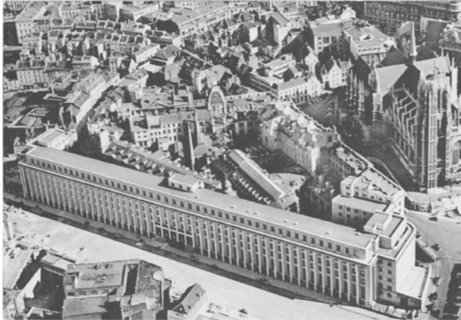
The first phase of the building(block on the Berlaaimontlaan) completed next to the existing bank
