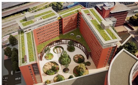
Figure 5.4: universe office building (Cerius Projects bv, 2022)
