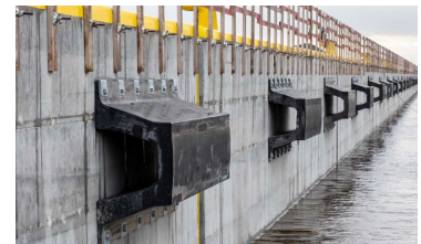
(b) Overview of V fenders on a quay wall [38]
