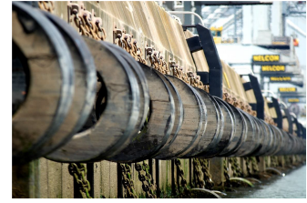
(b) Overview of cylindrical fenders on a quay wall [44]
