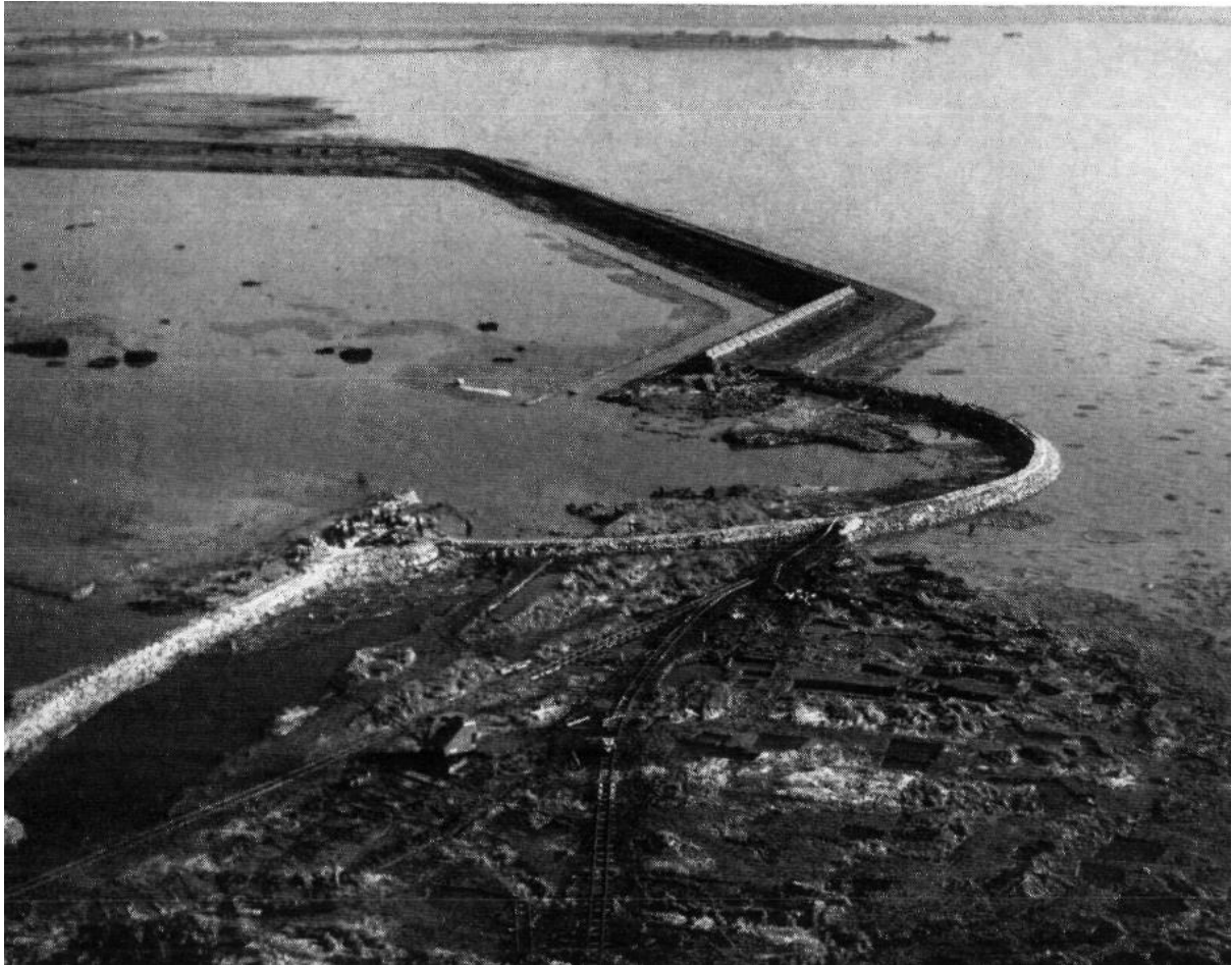
Figure 84: Elliptical erosion pattern in foreland after dike breach Note: reprinted from: "Verslag over de stormvloed", Rijkswaterstaat, 1961.
