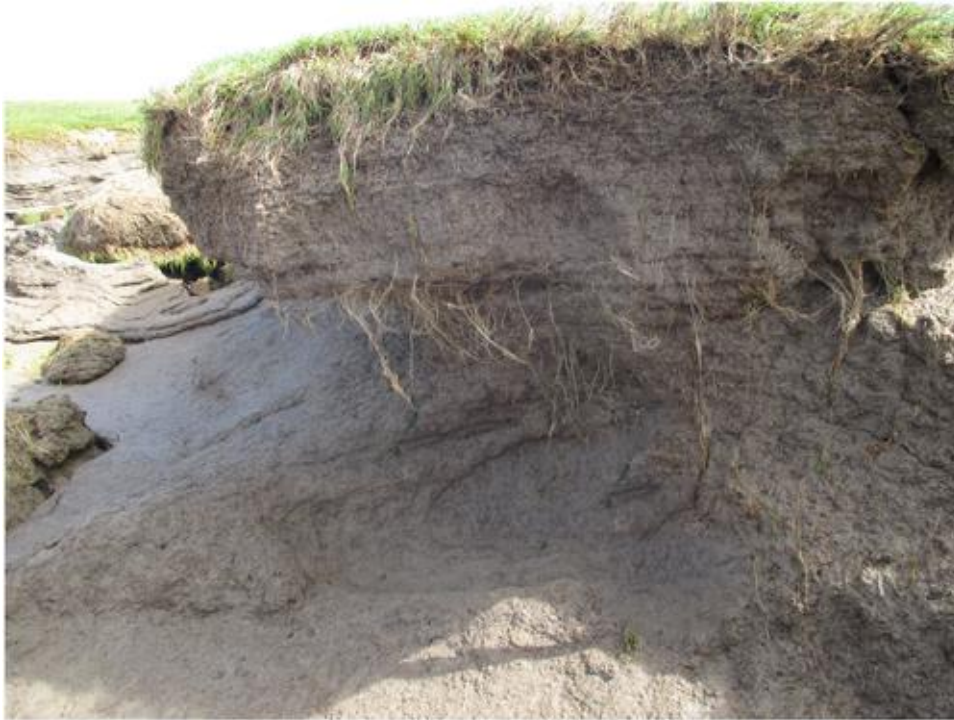
Figure 10: Foreland erosion restricted by system of roots
