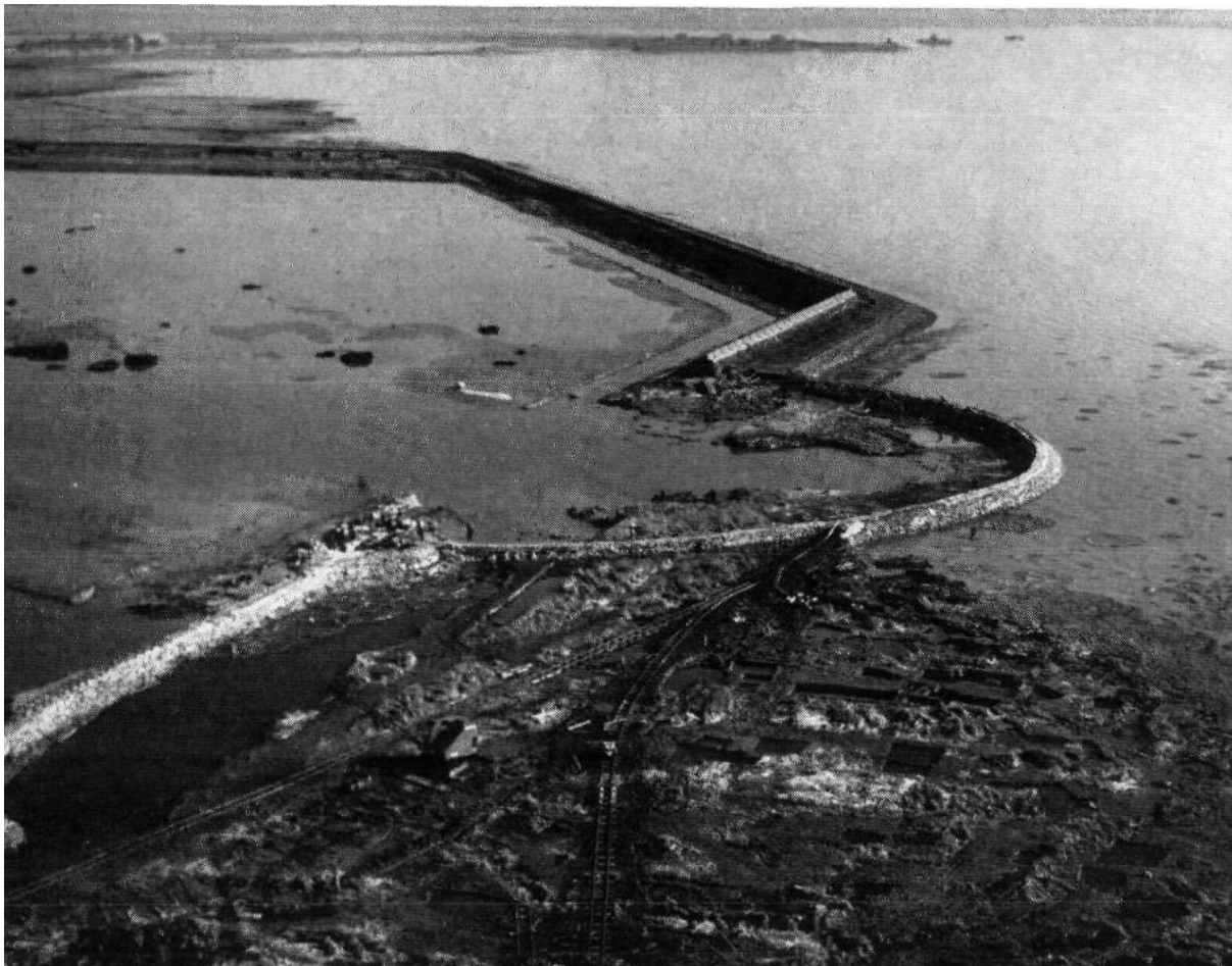
Figure 62: Elliptical erosion pattern in foreland after dike breach Note: reprinted from: "Verslag over de stormvloed", Rijkswaterstaat, 1961.
