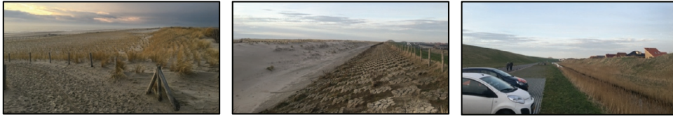
Fig. 2 Photo sequence of coastal flood defenses near Petten, the Netherlands. From left to right: seaward side of the Hondsbossche Dunes (left), back-dune fronting the dike (center), and backside of the dike (right). (Photos by J. Figlus.)
