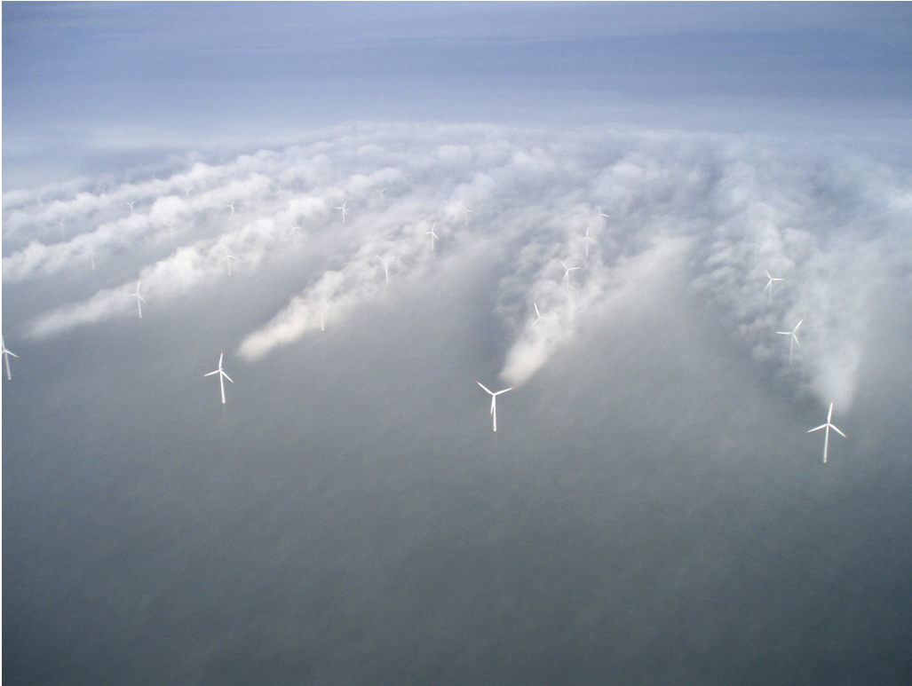
Figure 2.1: Wakes in the wind farm Horns Rev 1 [February 12th 2008]. (Owned by: Vattenfall. Photographer: Christian Steiness)
