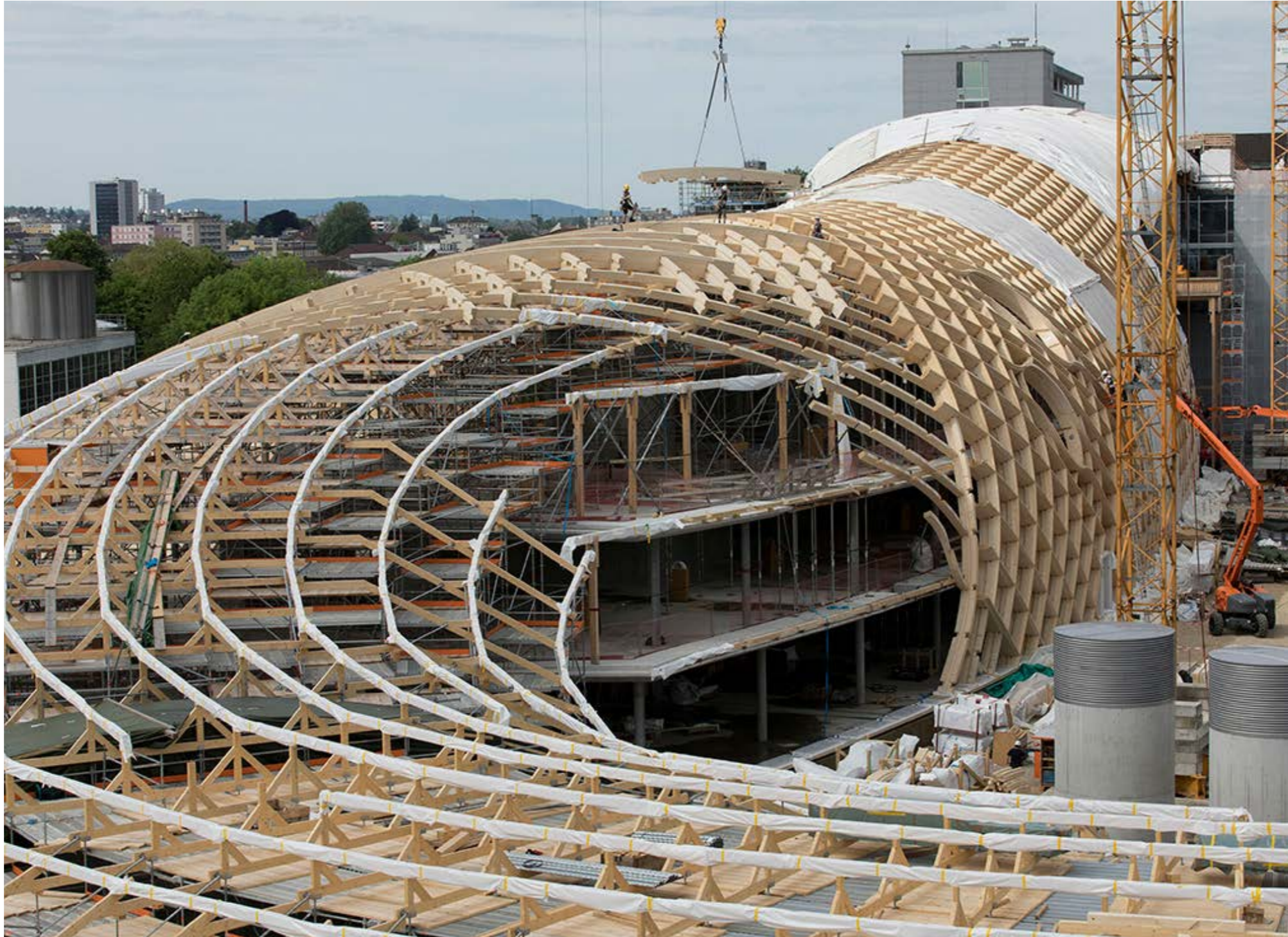
Building process Swatch Headquarters by Shigeru Ban
