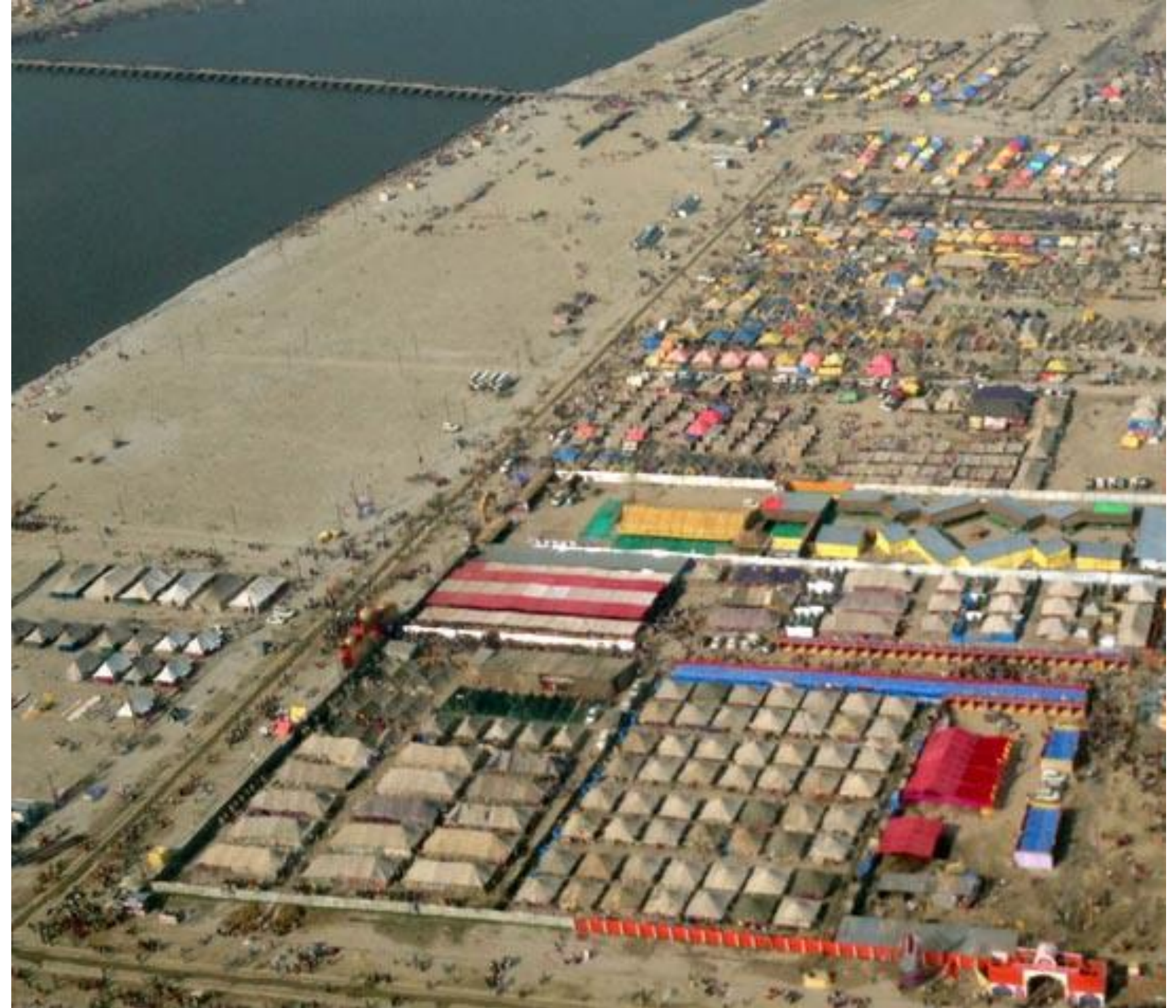
Delayed construction Management problems
