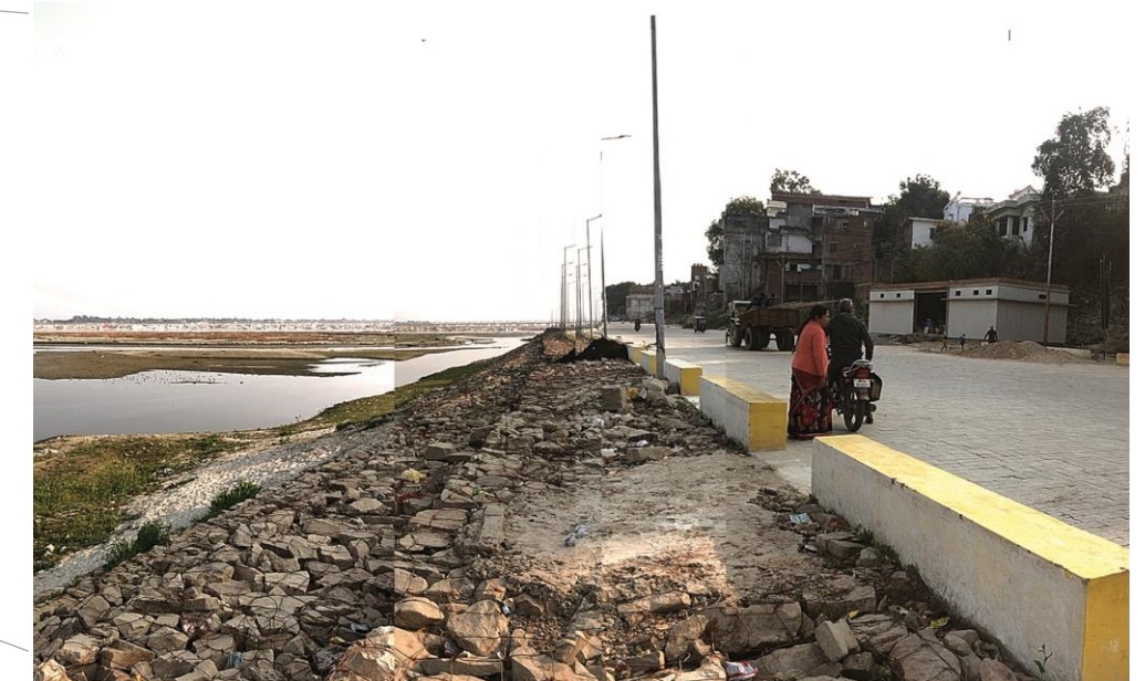
2 BUXI BUND EMBANKMENT
