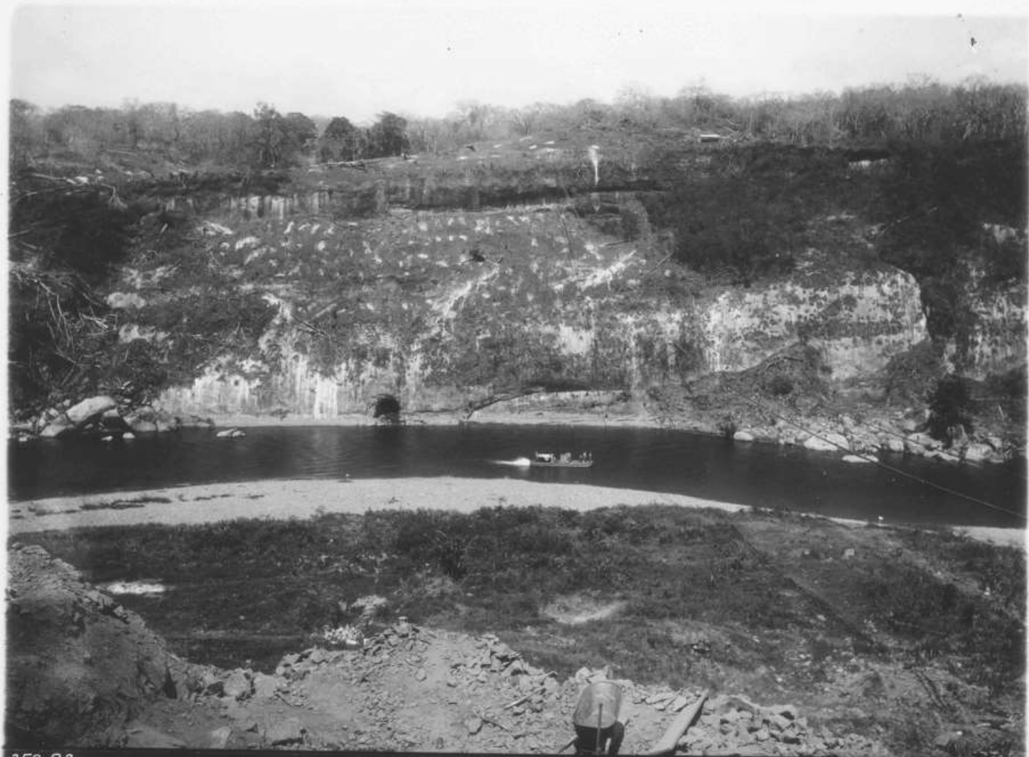
352-B 2 The Panama Canal. Madden Dam Project. View of Denuded Right Abutment and U.S. FRIGATE taking New Water Supply Pump to Intake. Taken from Point # 1-A. February 2, 1932.
