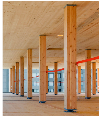
Figure B.8: Glulam beams and CLT slabs [37].
