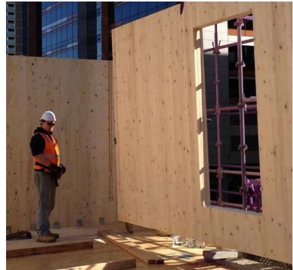
Figure B.4: Placement CLT with doorway already cut out [48]
