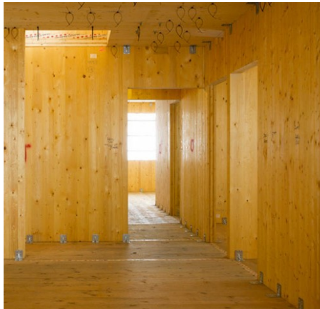
Figure B.2: CLT walls and floors Stadthaus [1].
