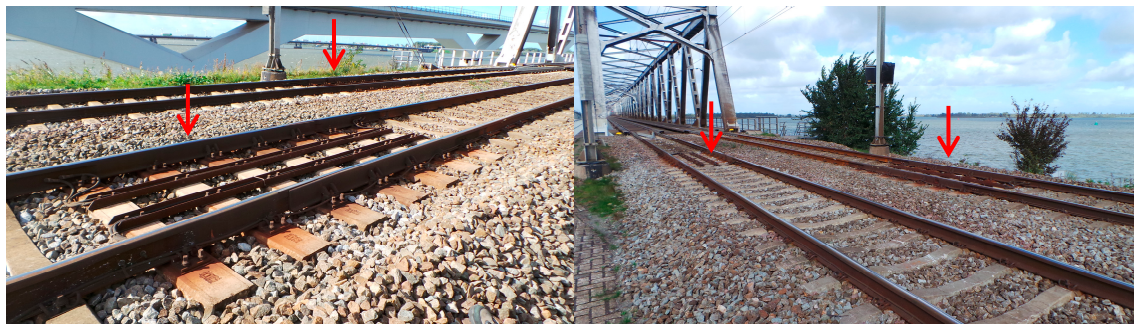
Figure 11. Expansion joints on the right side of the bridge.
