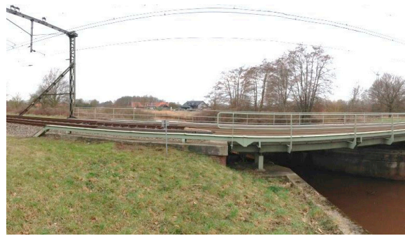
Figure 1. A typical track transition zone in the Netherlands.
