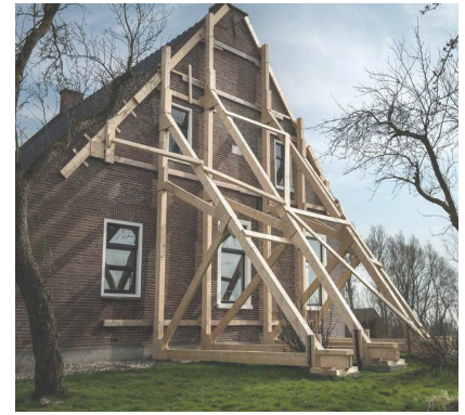
Figure 4: Auxiliary construction in Groningen
