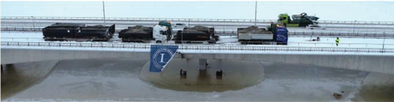
Figure 4. View of the midspan of the Kalix bridge under proof loading.
