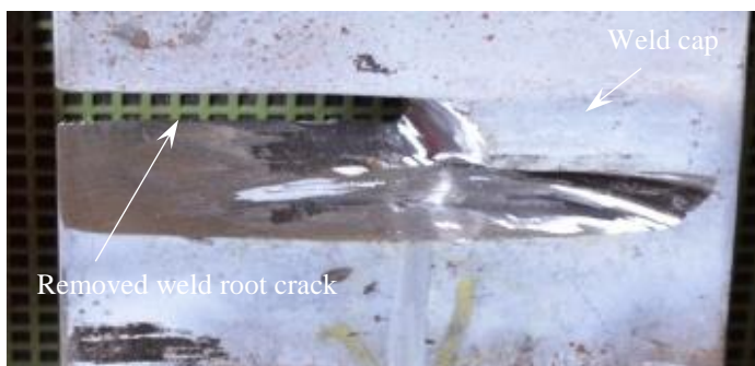
Figure 7. Removal of the crack at the weld toe of the weld root.
