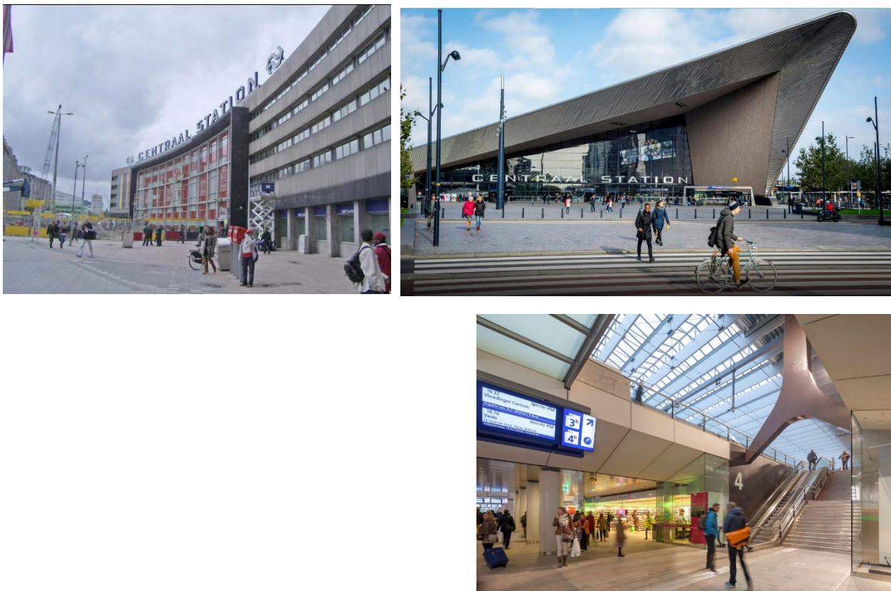
Fig. 7 Rotterdam Central Station (left old station, right new station)
