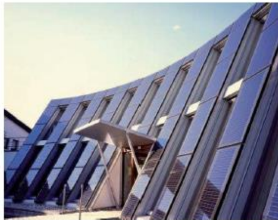
Figure 2.12 Integrated PV modules on a façade [18]
