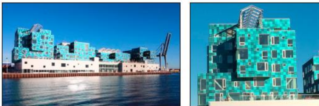
Figure 2.14 Copenhagen International School's (CIS) covered with Kromatix™ blue-green solar glass [19].
