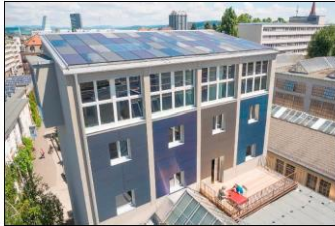
Figure 2.13 Coal silo building in Basel covered with colored Kromatix™ solar glass [20]
