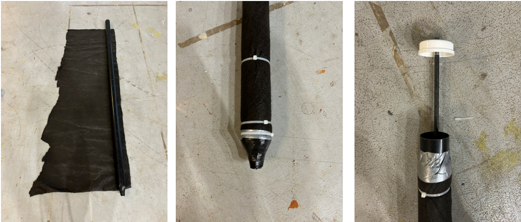
Figure C.4: Wrapping the well
