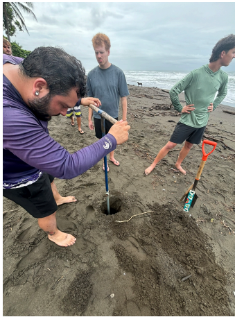
(a) Step 1: Drilling a hole for the well
