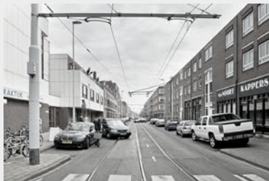
Figure 112: Zaagmolenkade, source: versbeton.nl (2013)
