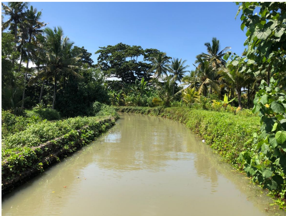
Figure A.9: View of the side channel
