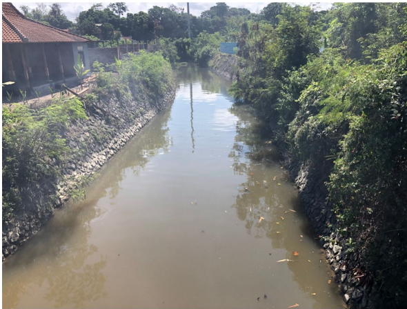
(a) View of side channel
