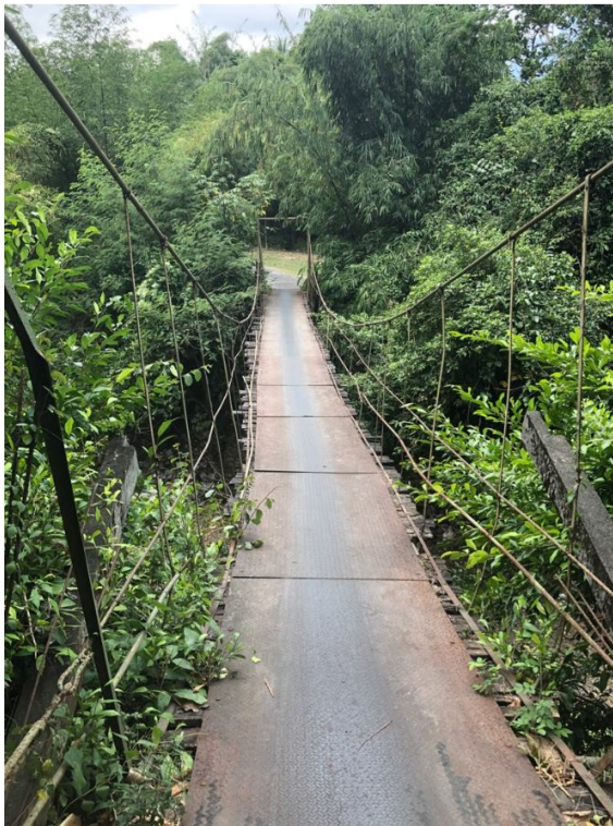
(c) View of bridge
