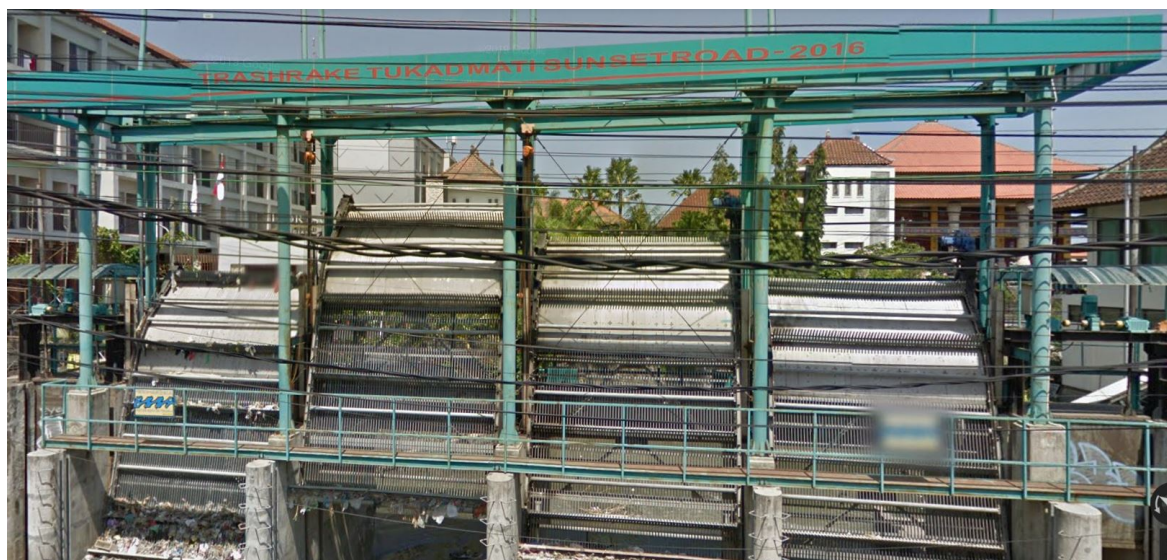
Figure 6.1: Existing structure 1 on river Tukad Mati (source:maps.google.com)
