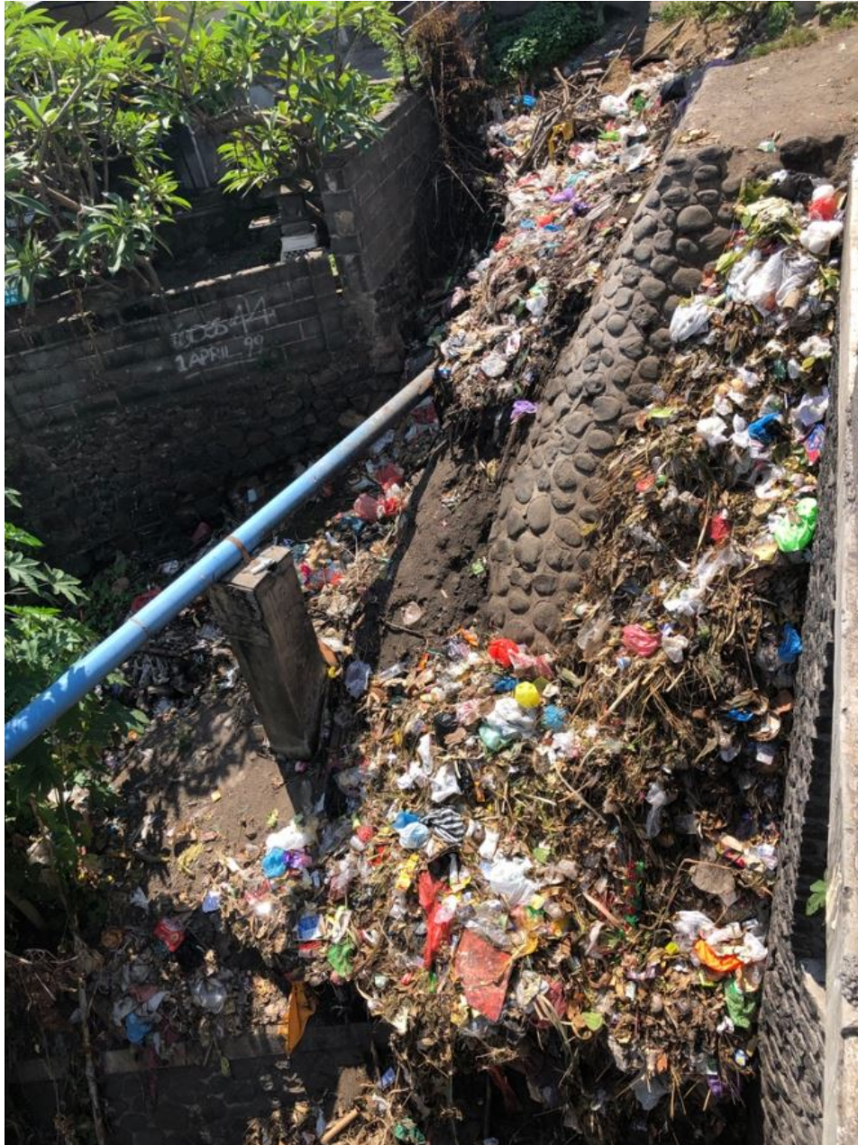
Figure A.28: View of the embankment
