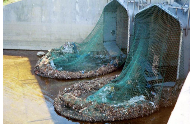
(b) Example of a drainage net system
