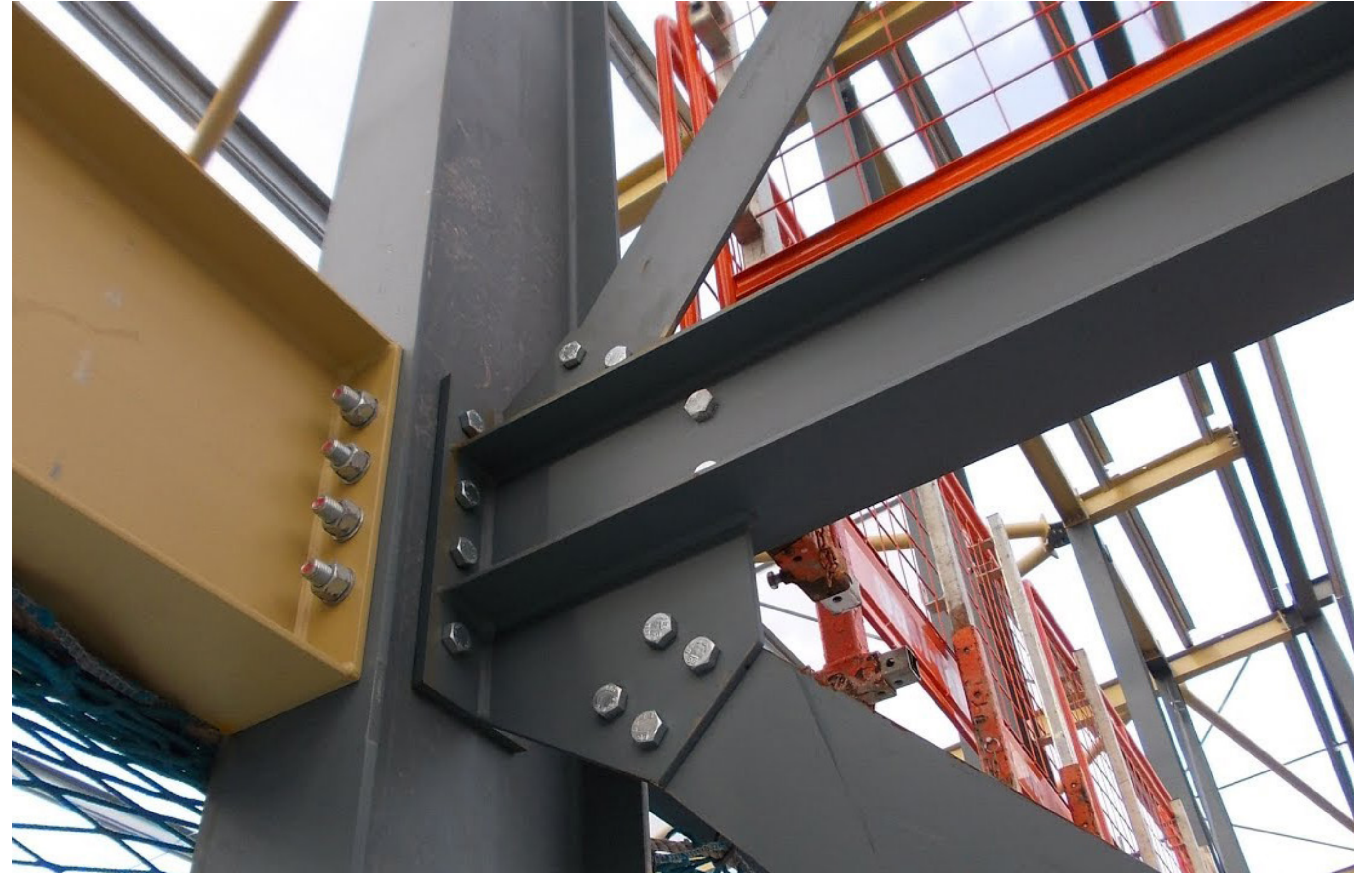
Image 8: Bolted Connections in Steel Structure (Rahman, 2020)
