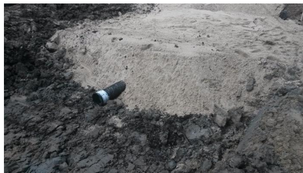
Figure 4.2: Photo taken during construction of the case-study bioswale
