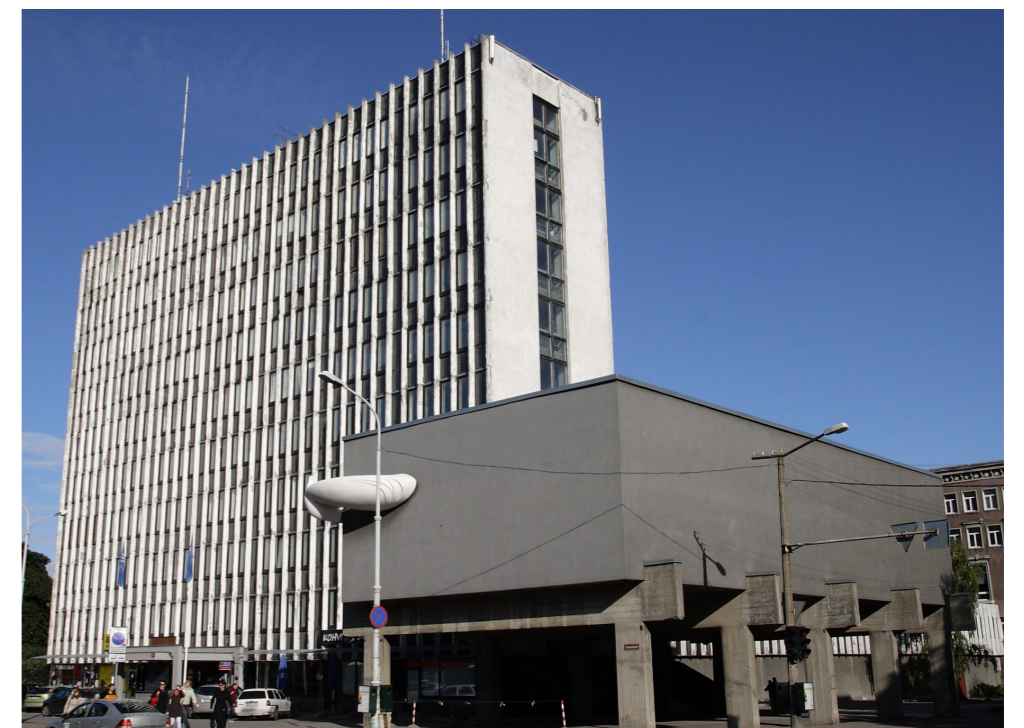
1972 New radio building + hall + passageway 2013 Facade repair
