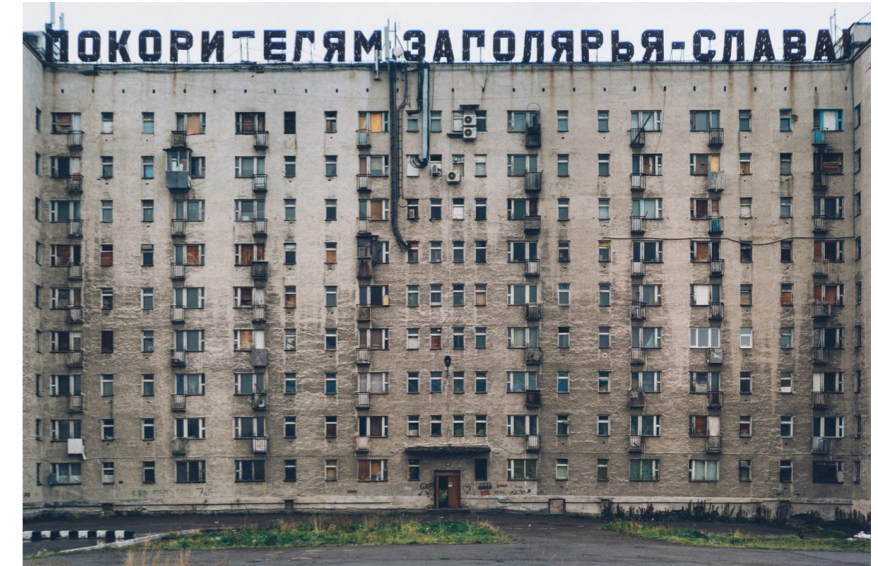
TP-8 type dormitory building, Vorkuta, Russia Photoed by: Arseniy Kotov
