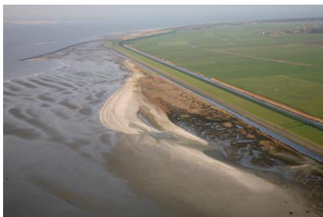
Figure 1. Example of a vegetated foreshore along a Wadden Sea dike in the Netherlands
