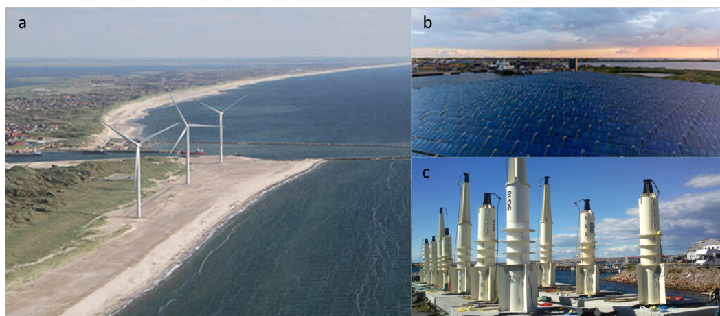
Figure 1. The RESs of Hvide Sande: (a) installed wind power park; (b) installed solar thermal park; (c) the wave energy converters used to form a wave power park.
