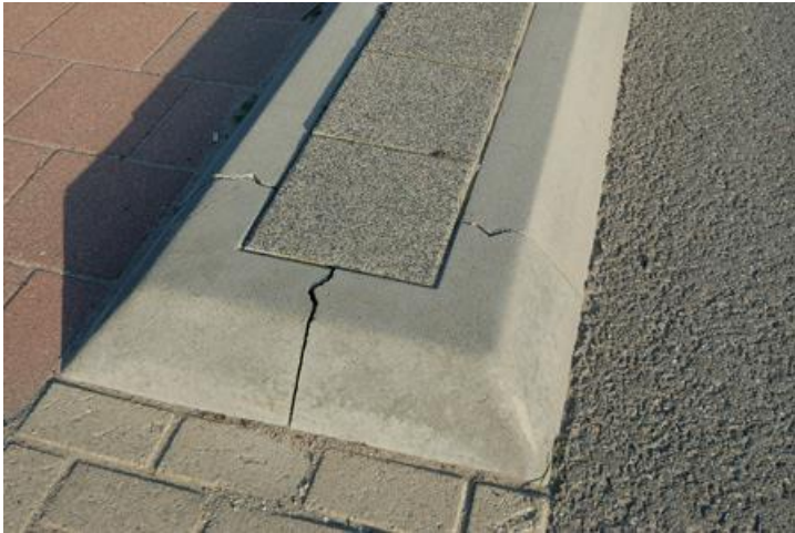
Photo from: struykverwoinfra.nl
