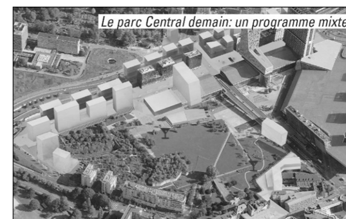
Figure 56: Euralille 3000 project attempts to improve city life by densification and mixed-used programming of station area (ma-geo)
