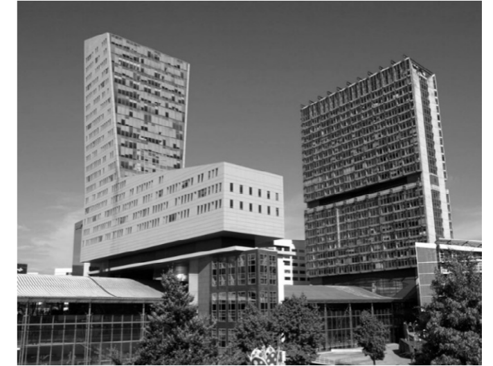
Figure 43: The Lille-Europe tower sitting on top of the Lille-Europe station designed by architects C. Vasconi and J. Burdese
