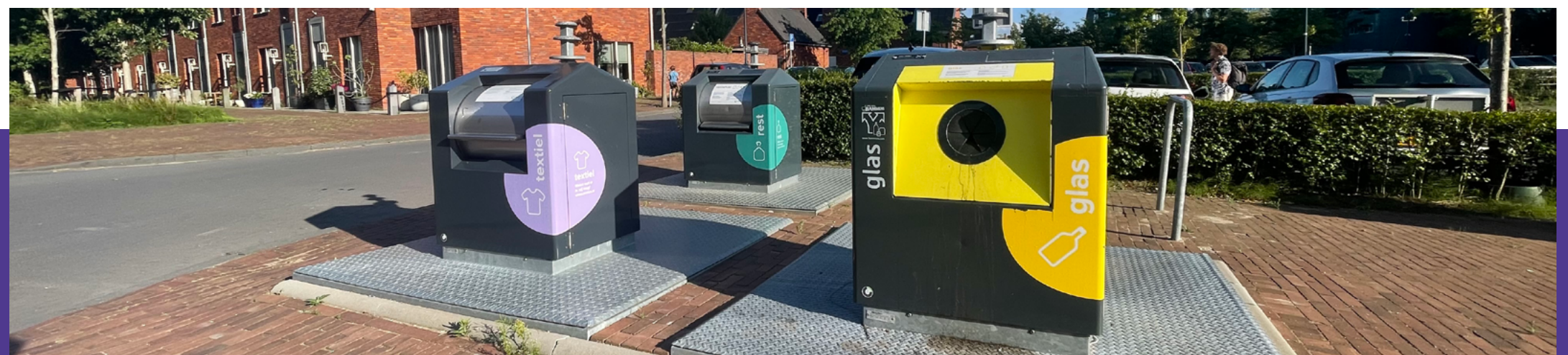
Figure 1.1.4. Picture of underground waste containers in the Netherlands
