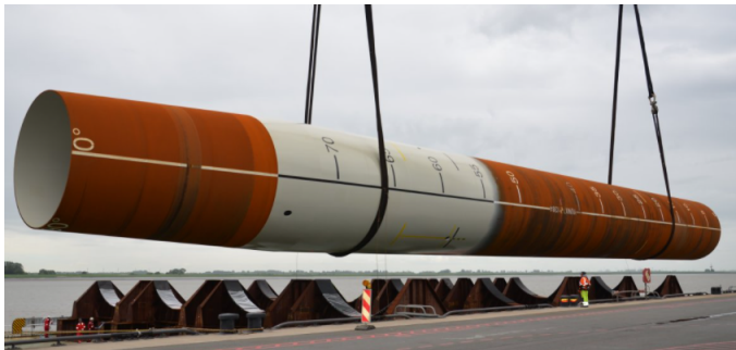
(c) Monopile loaded onto support points [50]
