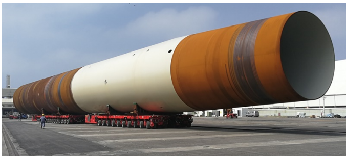
(b) Monopiles rolled out on SPMT's [49]
