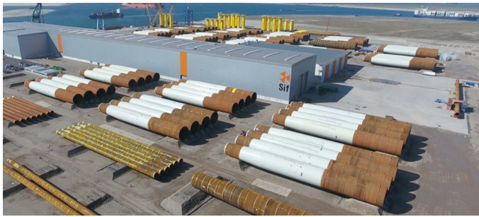
(a) Production site of monopiles and transition pieces at SIF on the Maasvlakte [3]
