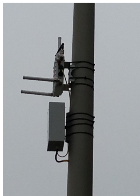
(b) Wi-Fi receiver mounted on a lamp post
