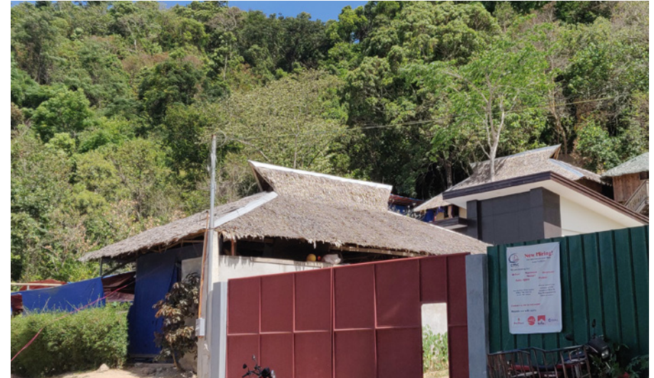
A building under construction, Palawan
