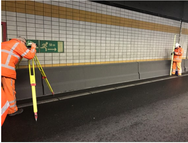
Figure 1.6: Tunnel settlement measured by manual leveling
