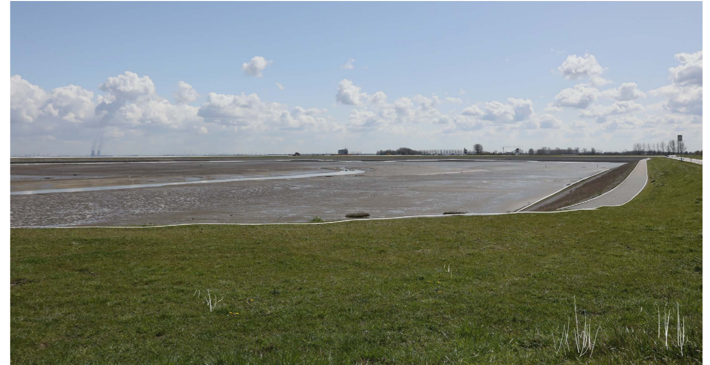
7.40.1 Impression of main dike at location of information centre(Author, 2021)
