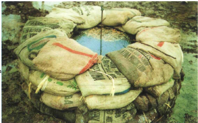
Figure 3.4: Ringing of a sand boil[20]
