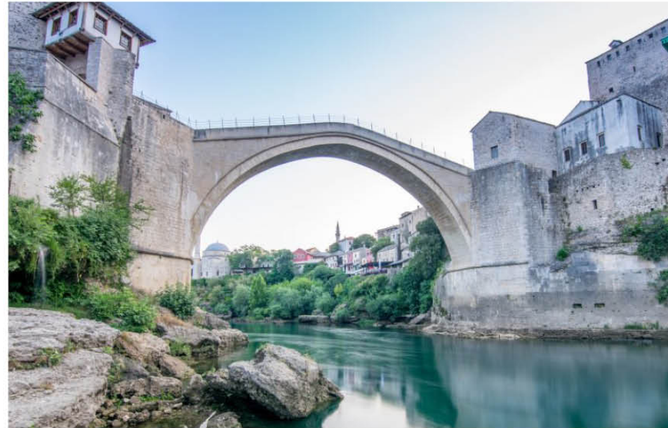
Old Bridge after reconstruction
