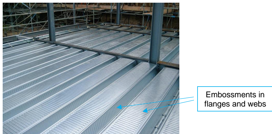
Figure 1.5 – Steel decking (ComFlor 210) is put in position between supporting beams[37]
