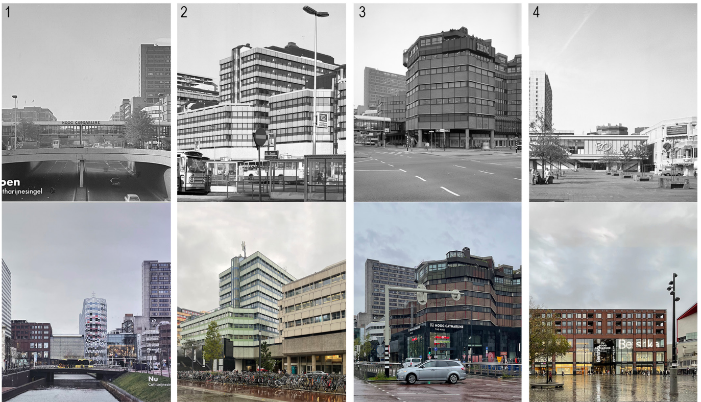
Fig. 8 Photo comparisons between the old and new facades
