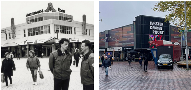
Fig. 3 Amsterdamse Poort simply used new facade panels to cover the old
