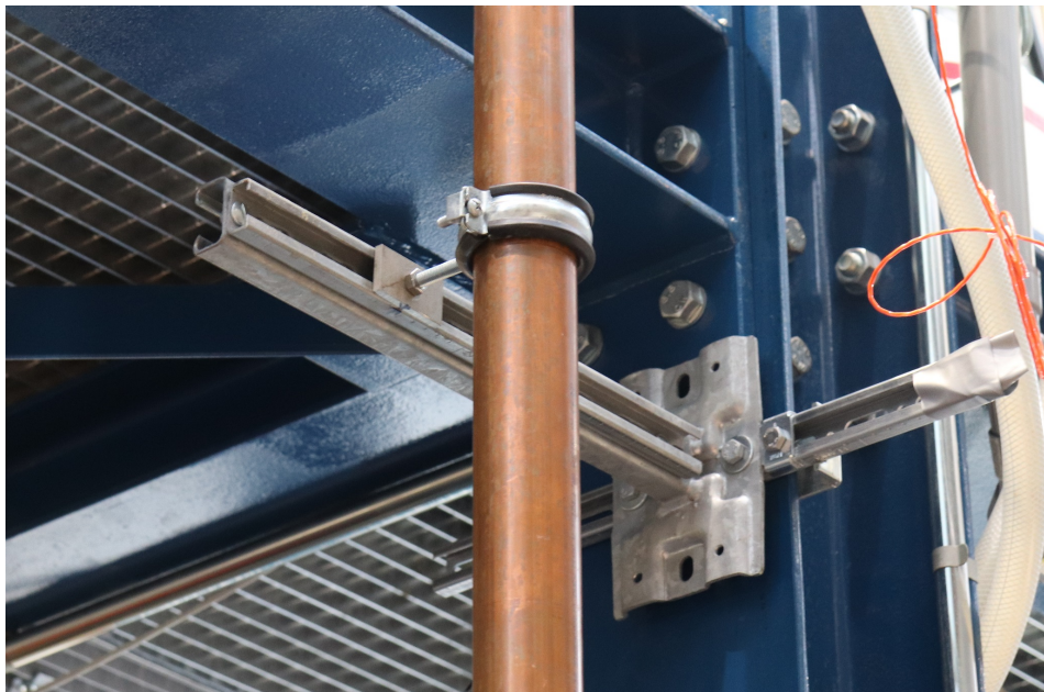
Figure 2.9: Clamping system to fasten the heat pipe to a frame.
