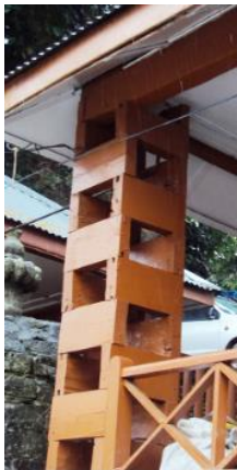
Figure 2.3: Thathara house : a) Thola columns, b) With stone masonry infill [21]
