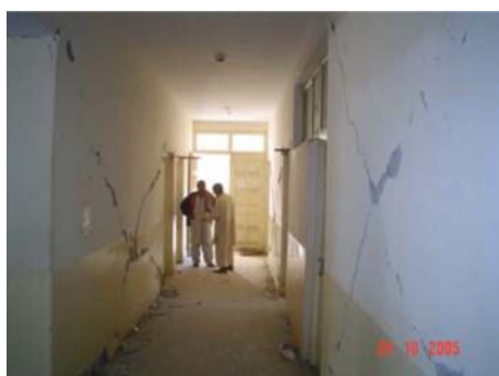
Figure 2.11: Diagonal shear failures of masonry piers [40]
