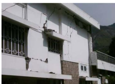
Figure 2.13: Horizontal flexural cracks due to rocking [40]
