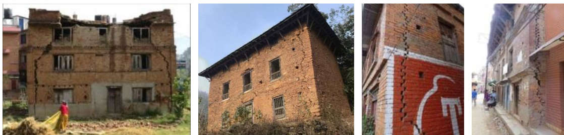
Figure 2.17: Separation of orthogonal wall [53, 54]
