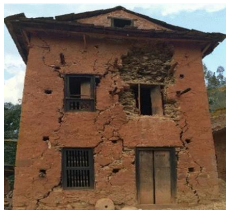
Figure 2.10: Diagonal cracks from openings [54, 55]
