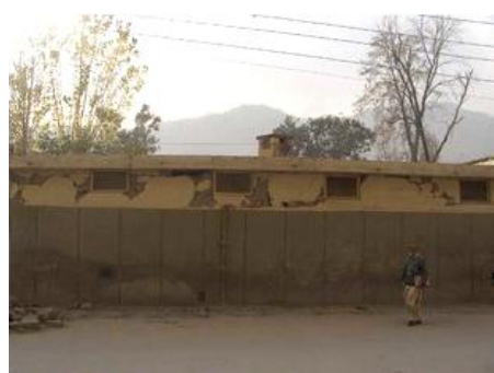
Figure 2.12: Damage due to multiple ventilators and openings below roof [40]
