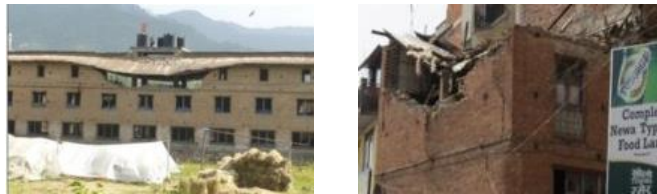
Figure 2.16: Inadequate connections to the diaphragm [53, 57]
