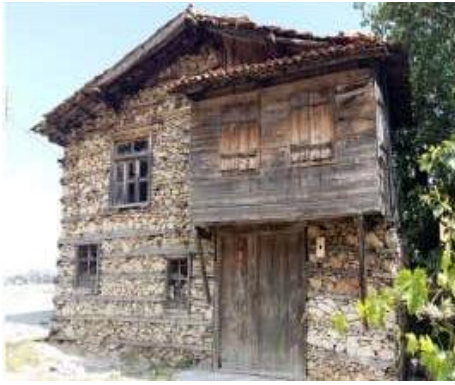
Figure 2.18: Timber-reinforced masonry : a) Ibradi button house in Turkey. Photo by Erarslan (2020), and b) Typical horizontal timber tie in stone masonry in Greek [61]
