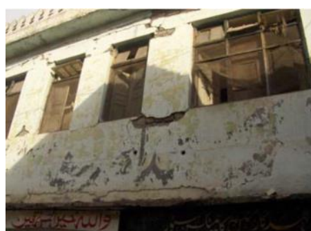
Figure 2.13: Horizontal flexural cracks due to rocking [40]
