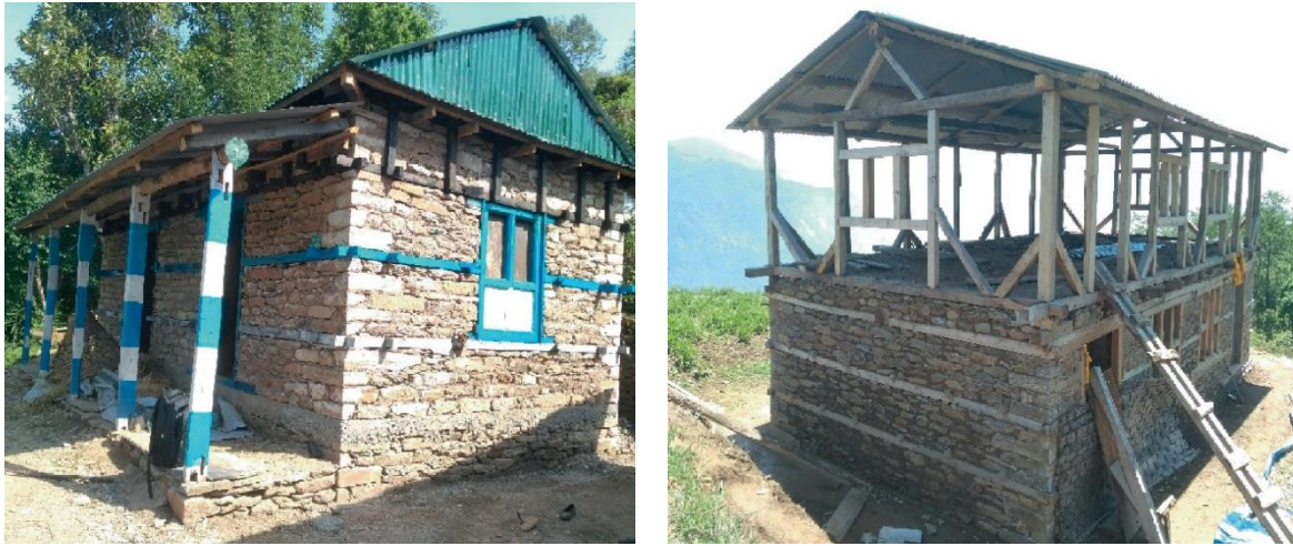
Figure 2.19: Stone masonry in mud mortar with horizontal timber bands observed after the 2015 earthquake in Nepal observed by [62]
