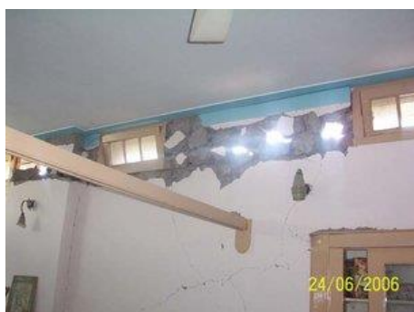
Figure 2.12: Damage due to multiple ventilators and openings below roof [40]
