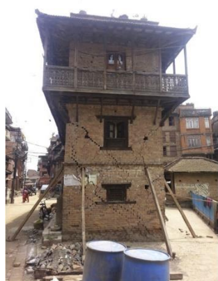
Figure 2.10: Diagonal cracks from openings [54, 55]
