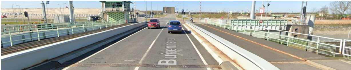
Figure 6.1, Oostsluisbruggen, deck view.
