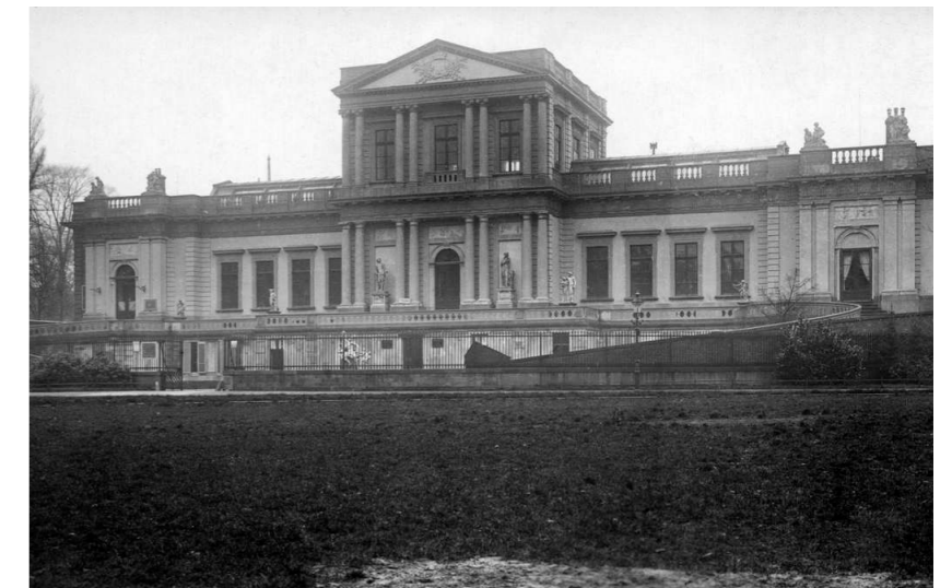
Figure 2.4 (Exterior of Paviljoen Welgelegen in Haarlem, 1913)
