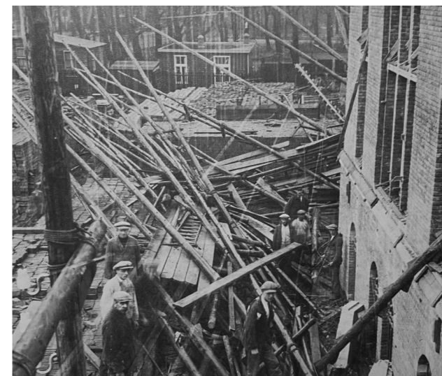
Figure 3.10 (Severe storm that damaged the scaffolding, 1921)
