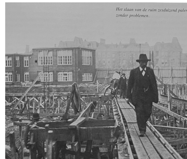
Figure 3.8 (The foundation work of 6111 piles, 1916)
