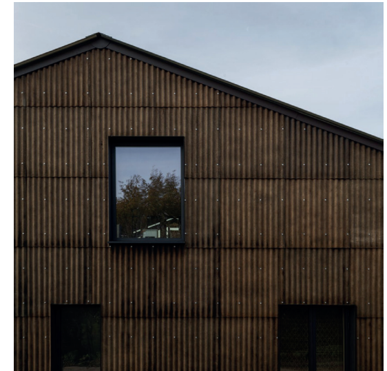
exterior hemp fibre corrugated sheets
