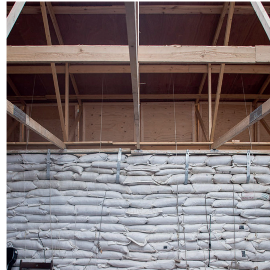
interior rice bags and timber structure
