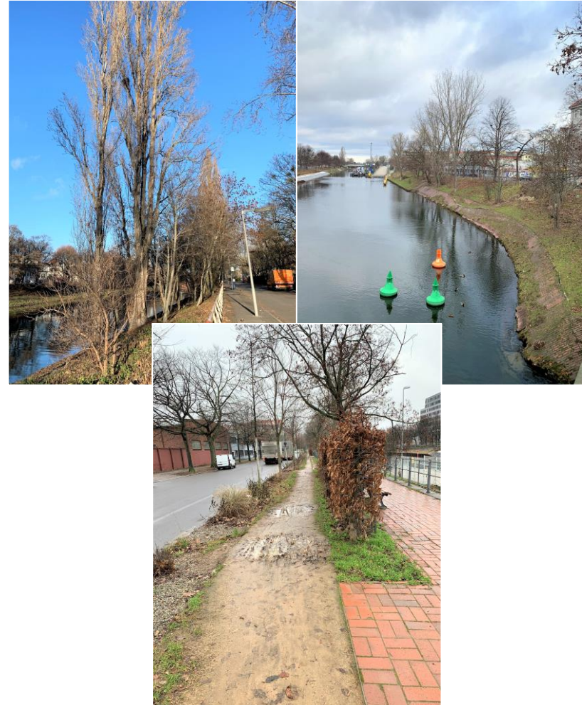
Status quo canal banks
