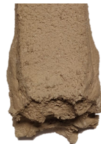
(d) Excess of material at beam end - top view
