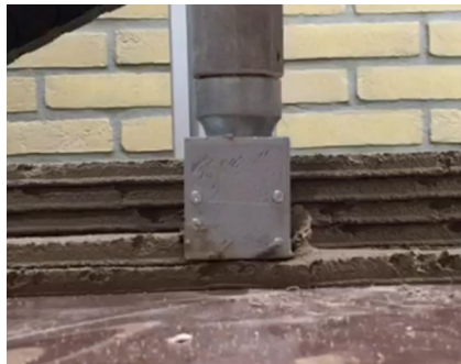
(a) Scraping and squeezing of the nozzle
