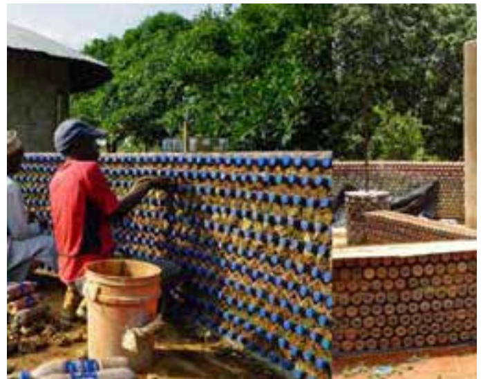
Figure 81 Construction with Plastic Bottles (Source : https://www.africanglobe.net )
