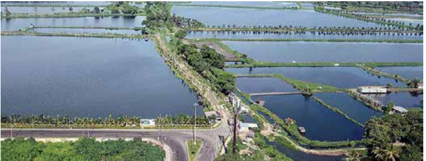
Figure 58 View of the wetlands ; Source : https://www.telegraphindia.com/states/west-bengal/plea-to-regularise-east-calcutta-wetlands-road/cid/1672879
