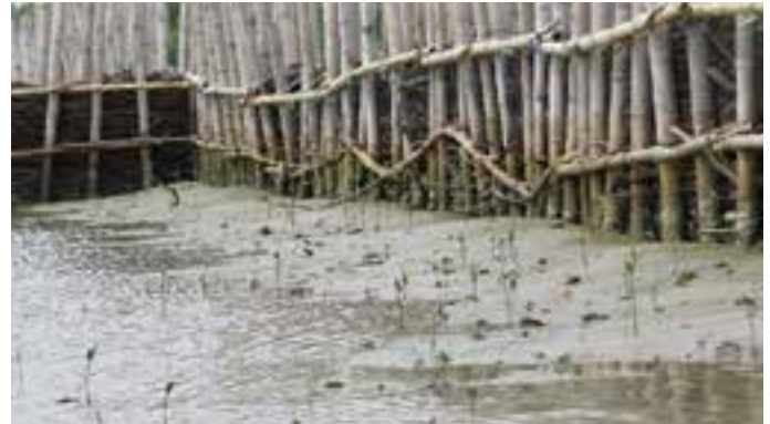
Figure 92 Growth of natural mangroves and sedimentation accumulation behind the location of Permeable Structures in Timbulsloko Village. Photo by Apri Susanto Astra
