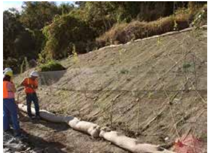
Figure 124 Example of a soft bank protection using anchored trees (SAFCA, 2019)
