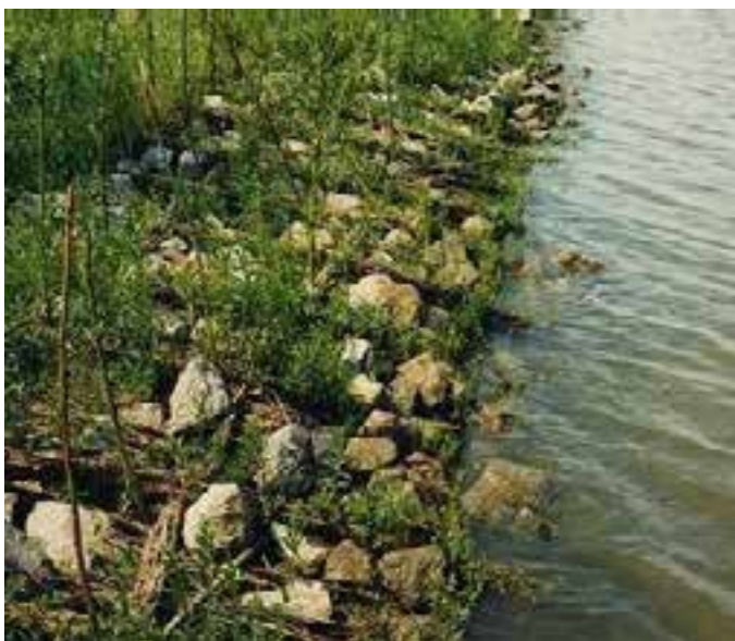
Figure 74 Example of a bank protection (Schierreck, 2012) (l), schematic overview of the reinforced mat (Schierreck, 2012) (r).
