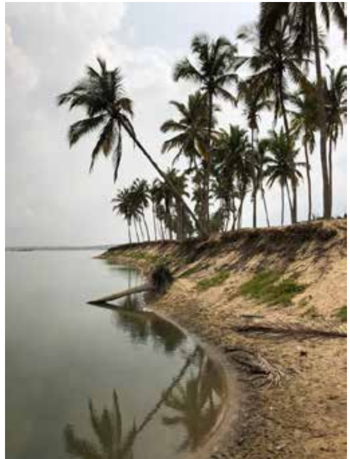
Figure 40 Erosion at the inner side of the lagoon
