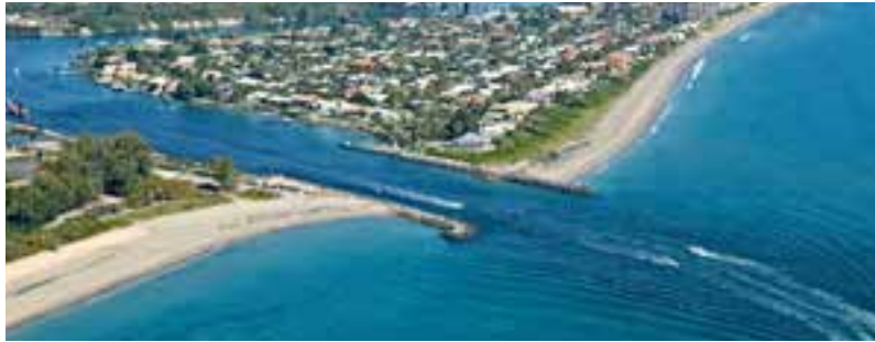
Figure 121 Tidal inlet including a bank protection (Sease 2019)
