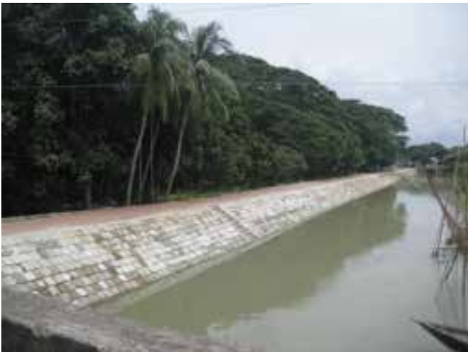
Figure 123 Example of a hard bank protection using rocks (Government of Bangladesh, 2019)
