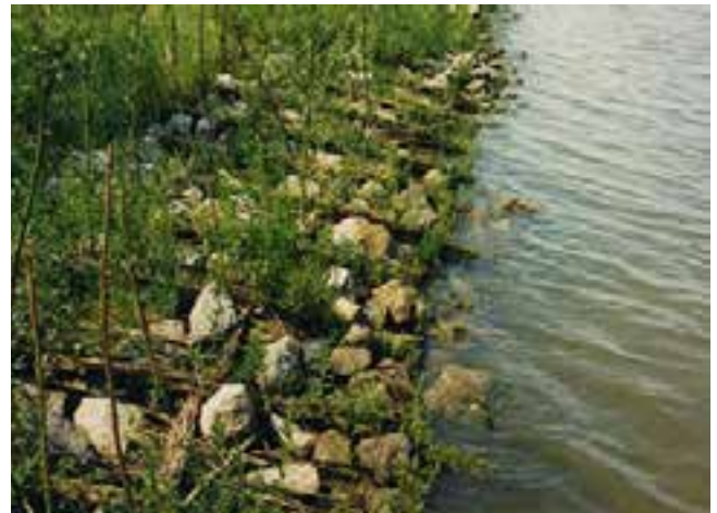
Figure 126 Example of a bank protection (Schierreck, 2012) (above), schematic overview of the reinforced mat (Schierreck, 2012) (below).
